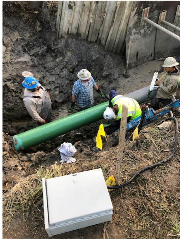
Pipe can be coated in Denso or other approved coating
