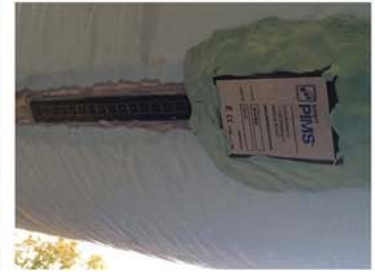
matPIMS™ 1x15 array permanently installed using viscoelastic putty to overcoat sensor strip and head before wrapping/backfill.
