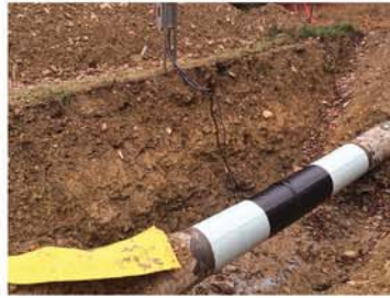
Fully coated and wrapped installation with RS-485 cable mounted in test station for data collection.
